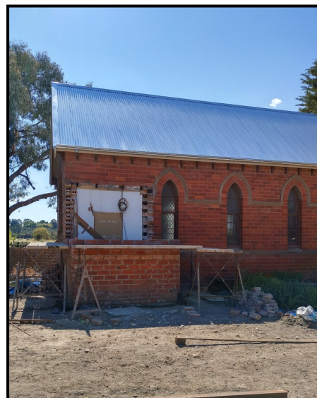
6. Rebuilding the sacristy.
