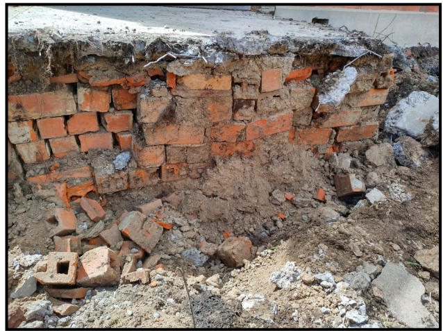
4. Bricks uncovered under porch landing.
