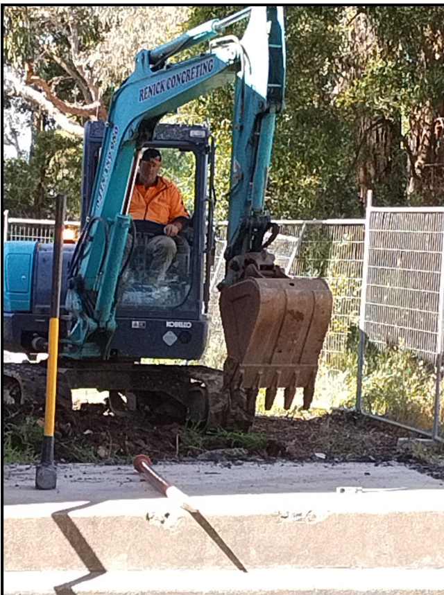
9. Preparing area for new access ramp.
