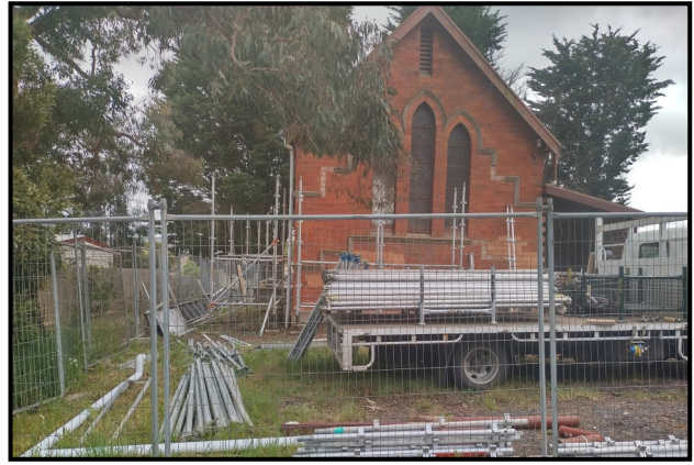
2. Scaffolding ready to be erected.
