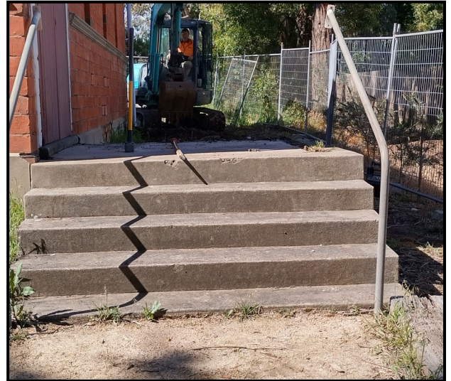
8. Steps being removed for the new access ramp.
