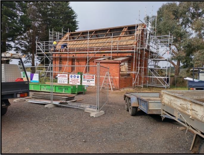
7. Roof being removed
