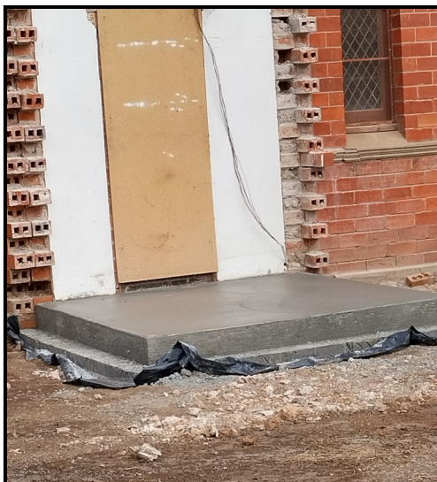
5. New sacristy floor laid.
